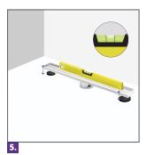
Place the drain leveled in all directions by regulating the metallic feet and using the leveling ruler to guide you.
