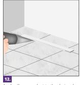
Apply silicone sealant to the drain edge, covering the joint properly, to guarantee proper fixation and waterproofing.
