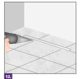
Apply silicone sealant to the drain edge, covering the joint properly, to guarantee proper fixation and waterproofing.
