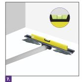
Pour the mortar mix into the bottom area of the drain base to provide support and guarantee the leveling.
